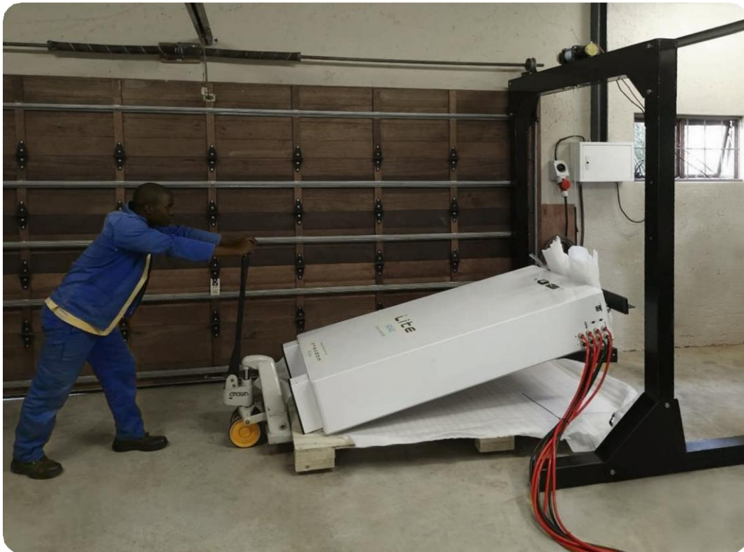
Fig 3.5 Site Assembled Gantry with Electric Hoist
