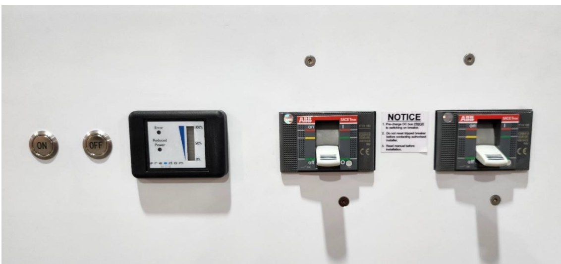
Fig 11.1 “ON” and “OFF” Buttons – Breakers shown in OFF position
