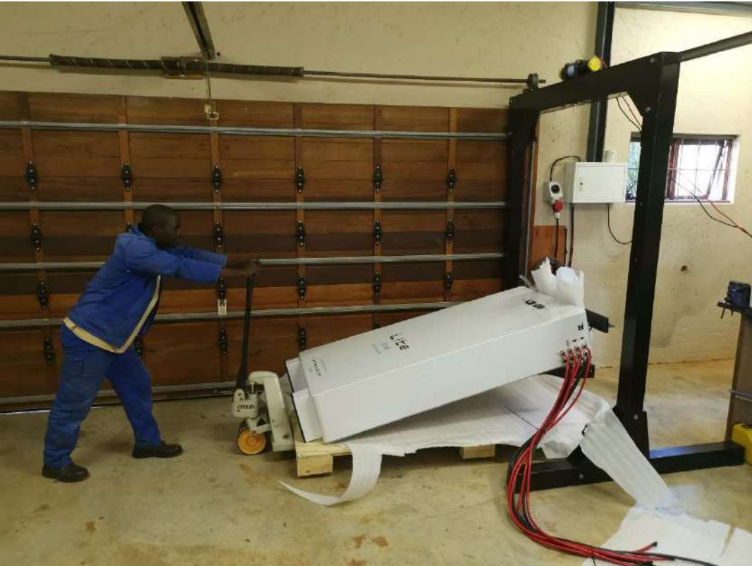
Fig 3.5 Site Assembled Gantry with Electric Winch
